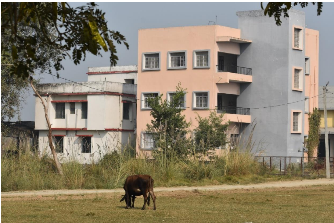
Image 88 : Other Govt. Constructions On Raghopur Diara [Vaishali District]
