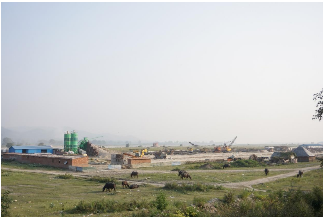
Image 65 : Construction Activities On Bairagi Camp Island
